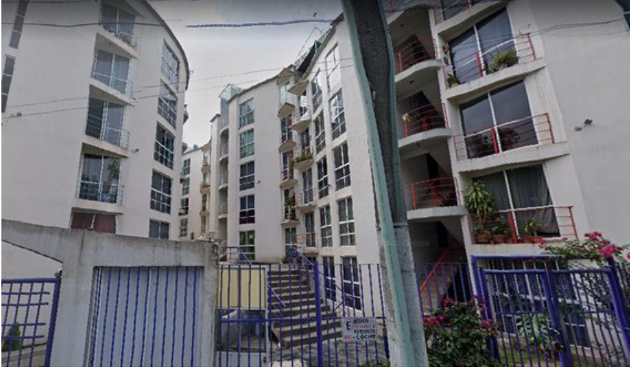
Figure 13. Guendaliza'a Cooperative. Source: Google Street View.
